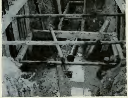
The drainage system
